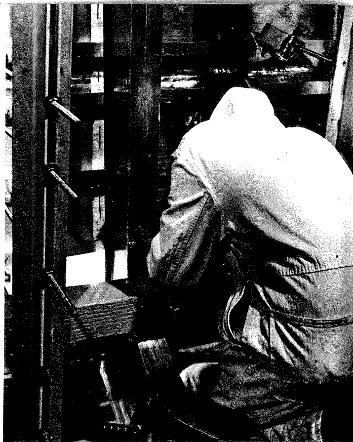
Aluminum plates being shaped to the ship's ribs. The novel system of turnbolts seen here was used because the hull was stressed. This was exacting work that had to be done in correct sequence, for otherwise the plate would buckle rather than bend. Author's photograph, copyright.
